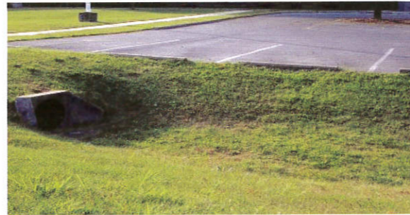
(Dry Swale to help absorb parking lot run off)
